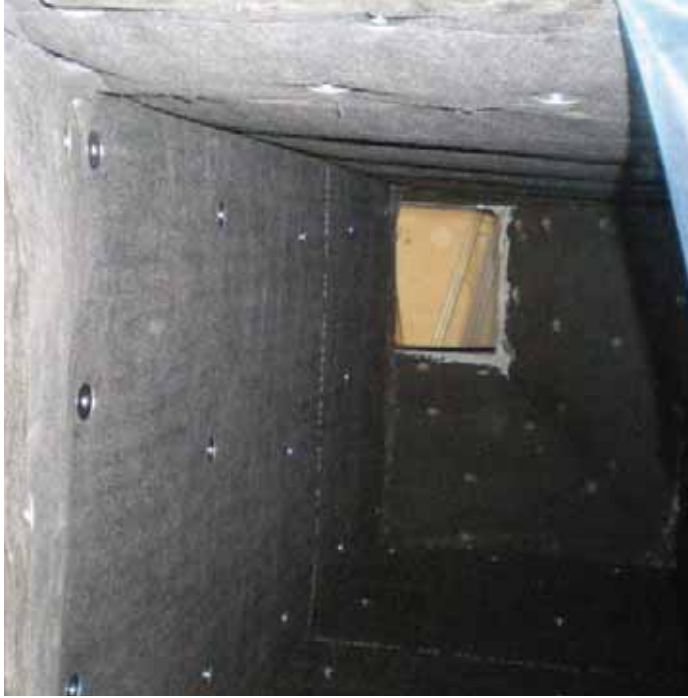
Glass fiber (shown left) is the most commonly used material for duct liners. It is manufactured in flexible batts and rigid boards. Glass fiber ductliner (top right) usually has a black coating.
